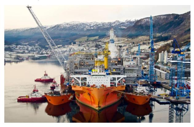
4. Topside float over installation with the tip of the SPAR hull above the waterline in between the S-class vessels (© Espen Rønnevik/Boskalis):
