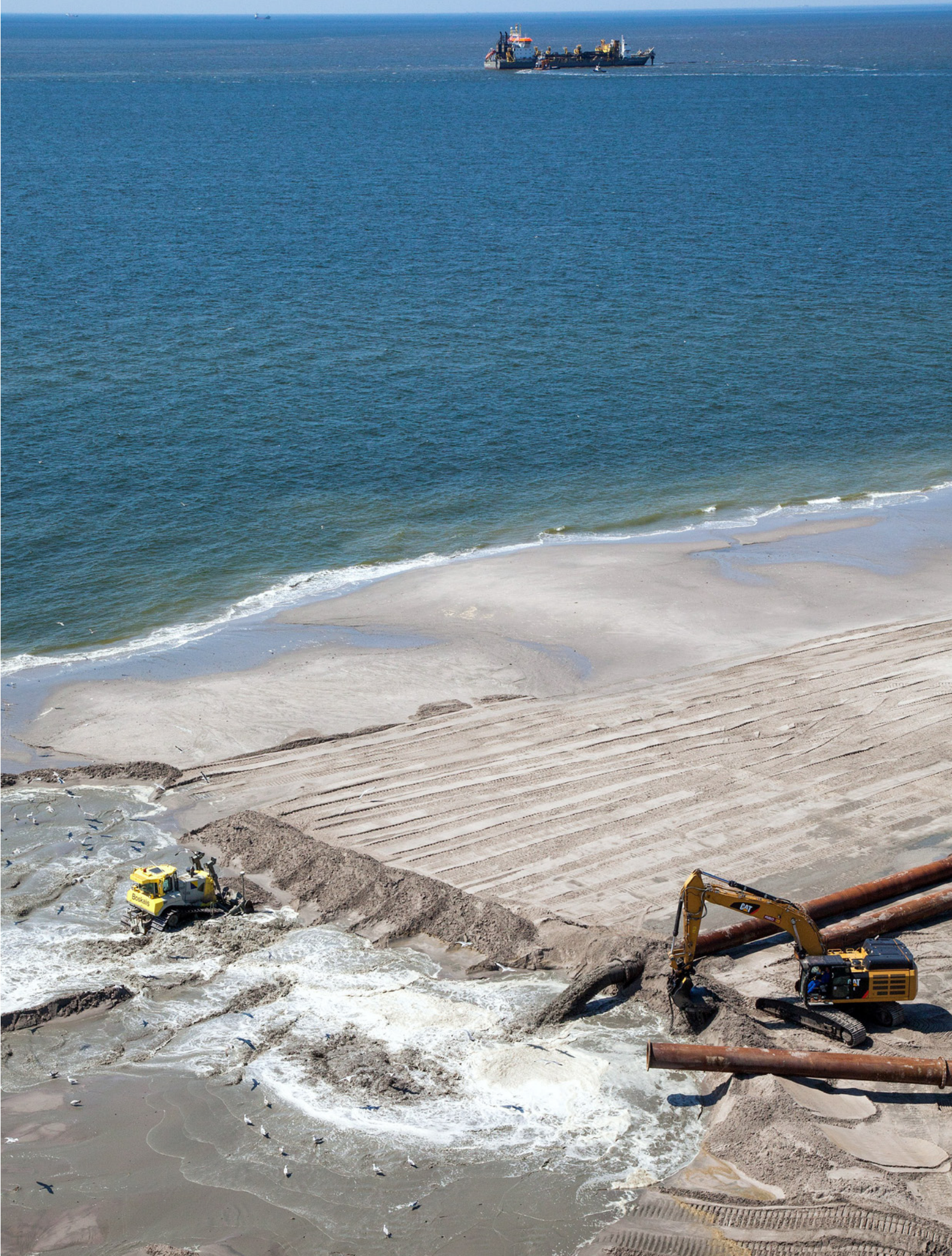
Maintenance work at Maasvlakte 2 in Rotterdam
