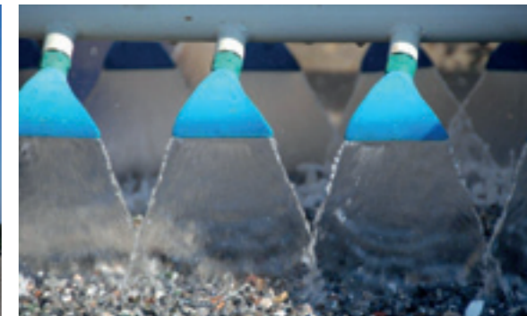
top middle TORONTO, ONTARIO, CANADA Construction of the Mobile Soil Washing Plant, for the Toronto Soil Recycling Demonstration Project.
