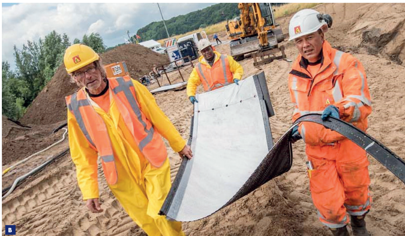
A The cassette in the dyke body B The geotextile
