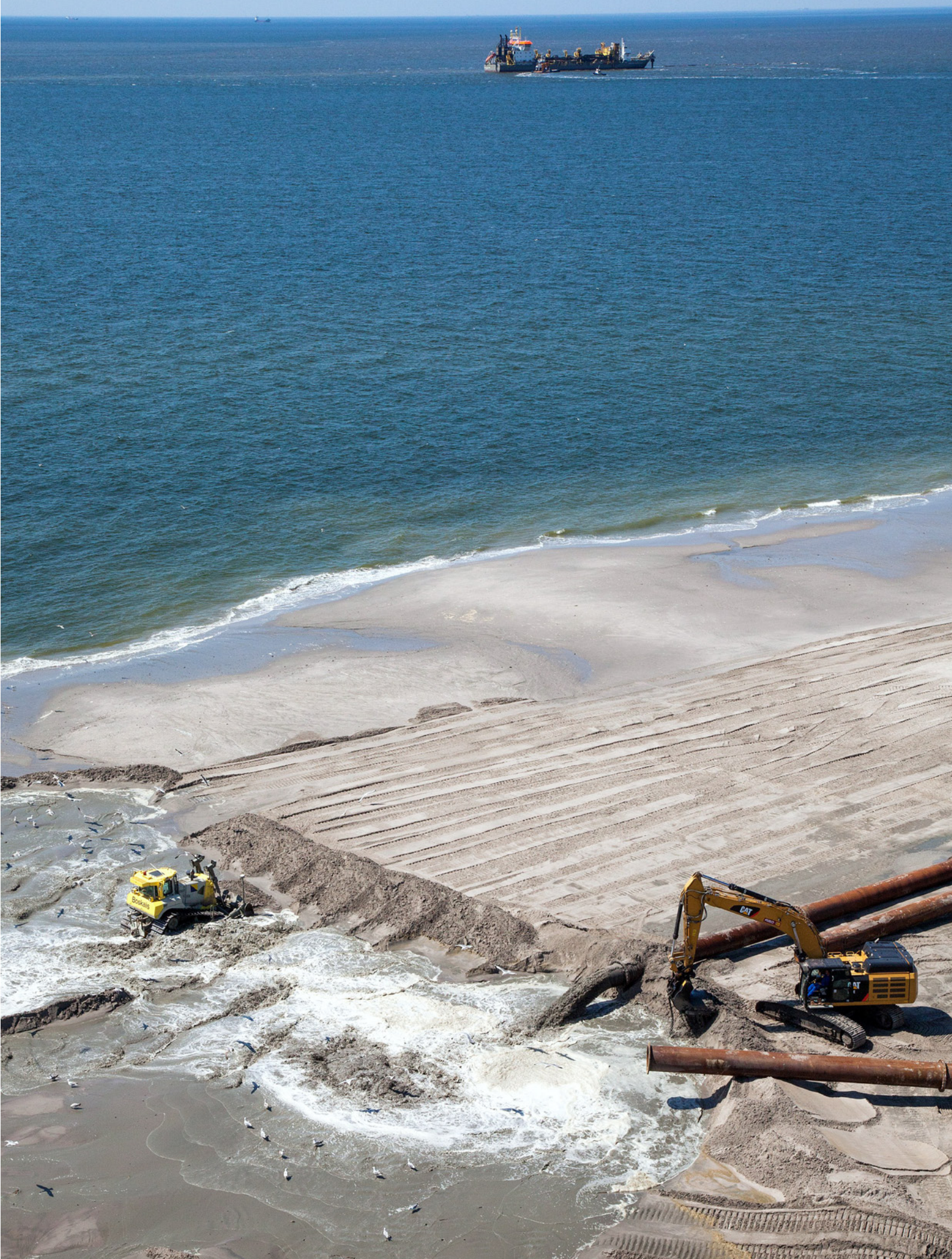
Maintenance work at Maasvlakte 2 in Rotterdam
