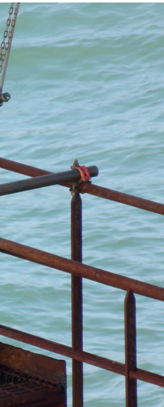
Riser clamp installation by rope access.
